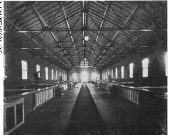
MECHANICAL FILTER PLANT, ERIE, PA.
